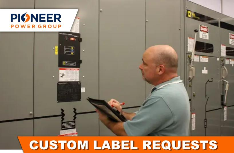
Pioneer Power Group was contracted to perform an arc flash study and to provide arc flash labels showing relevant incident energies. The customer had specific, unusual requirements for the layout, text, and colors on their arc flash labels. Over the course of several projects for this customer, we modified the labels to match what was required for their specific purposes.
